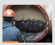
Steel cylinder and concrete wires exposed
