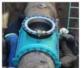
Mechanical joint line-stop fitting installation
