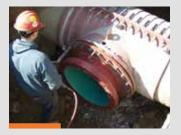
Gland installed and sleeve pressure-tested
