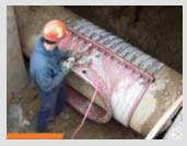
Sleeve grouted and tightened around pipe
