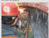
Cutting torch removes reinforcing steel wires
